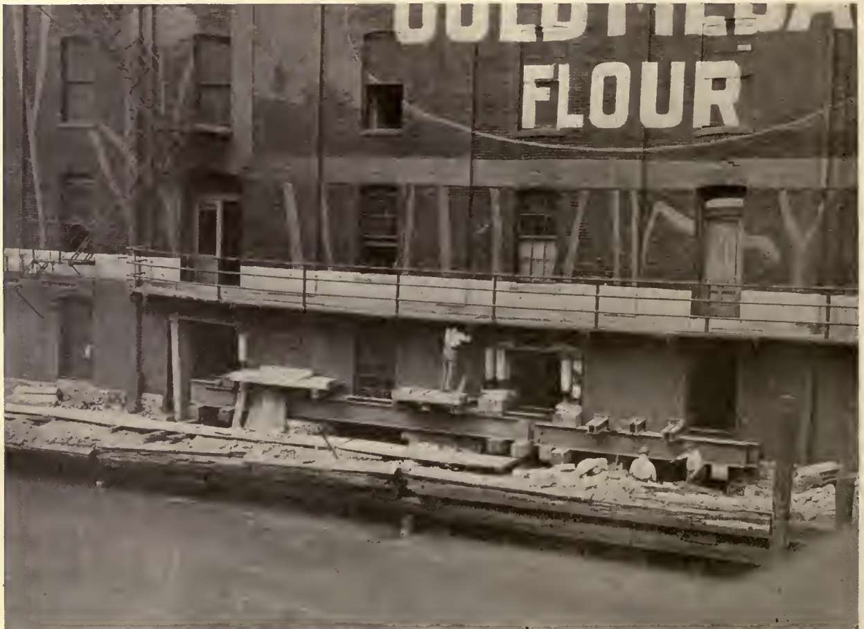
THE CENTRAL WAREHOUSE, CHICAGO Showing the method of raising and supporting the wall during the reconstruction of the foundation
